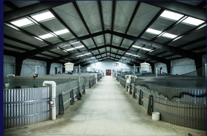
Recirculating aquaculture facility
